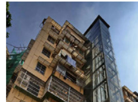
Modernization and Upgrading
