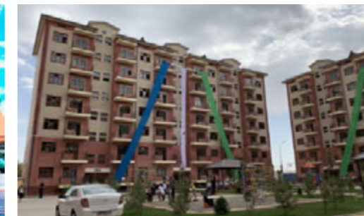
Government affordable houses (Uzbekistan 689 units)
